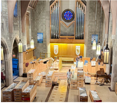
This pipe organ that once stood in a Richmond church is currently being refurbished by C.A. Zimmer Organ Builder to fit First Baptist.
